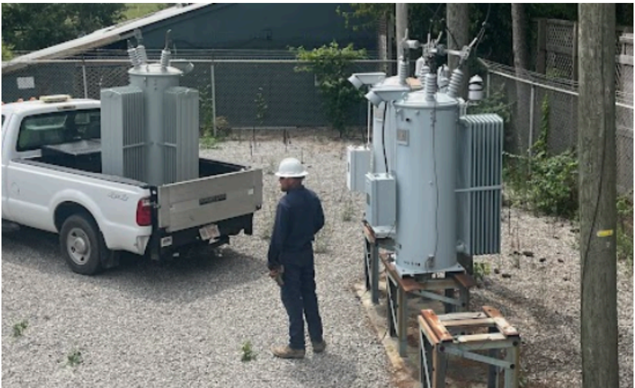
Recent electric department project at the new Center Circuit build.
